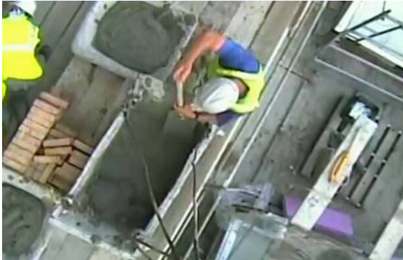
View from Crane Operator's Cab
