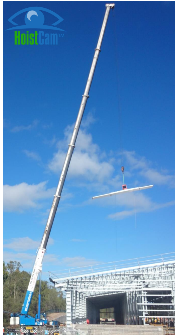
Figure 2. Positioning Roofing Panels with Telescopic Boom Crane.
