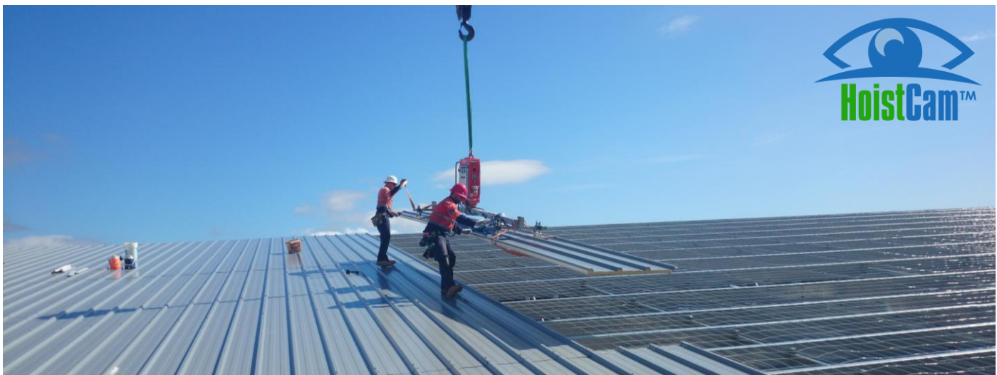
Figure 1. Positioning and installing insulated roof panels.
